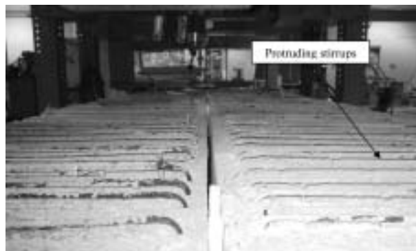
Fig. 9—CFCC shear stirrups protruding from box beams of Bridge Model BBC-I.
