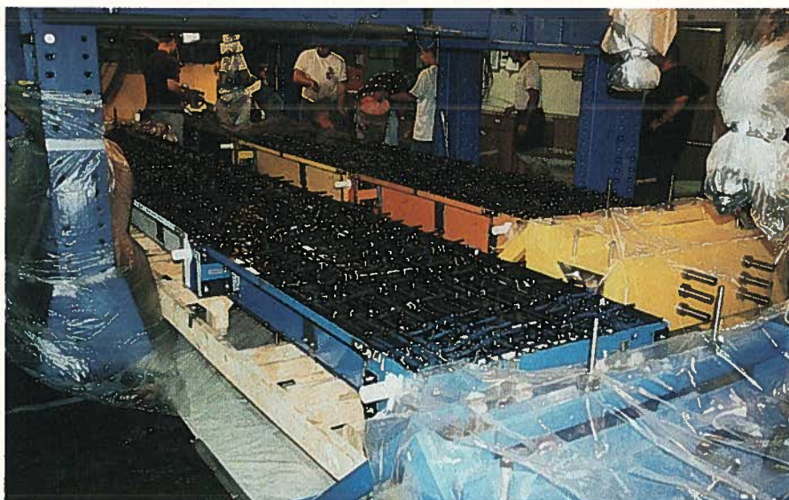
Fig. 9. Girders CDT2-1, 2 prior to casting concrete.
