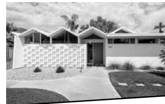
1960-70s+ - folded metal; invented precast concrete
