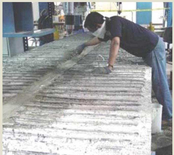
Figure 13. A graduate student fills the gap between adjacent box beams of a bridge model with concrete.
