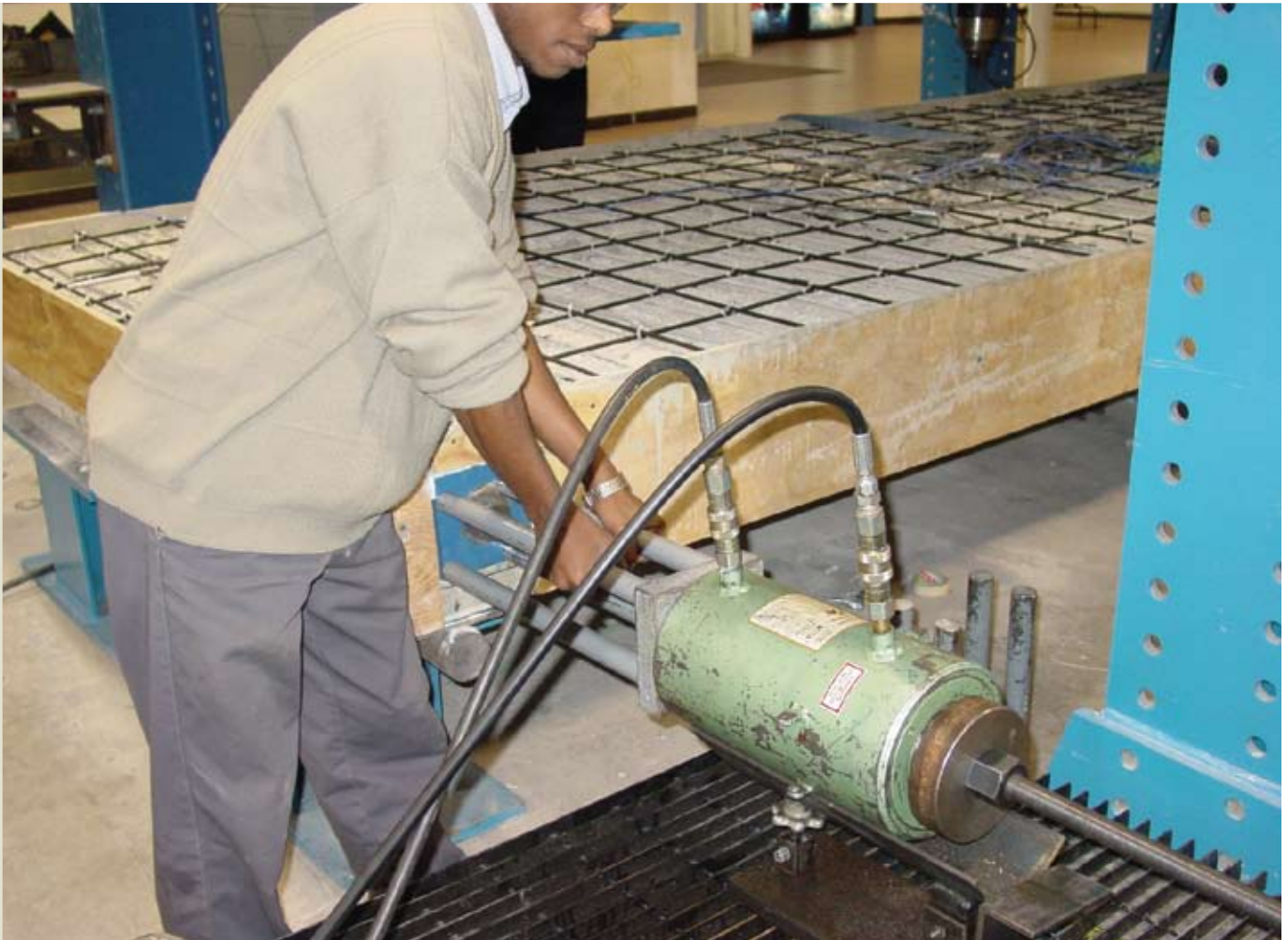
Figure 14. A bridge model receives an initial transverse post-tensioning force, which was necessary to maintain the structural integrity of the two adjacent box beams and to prevent any differential movement during longitudinal post-tensioning, casting of the deck slab, and application of external loads.
