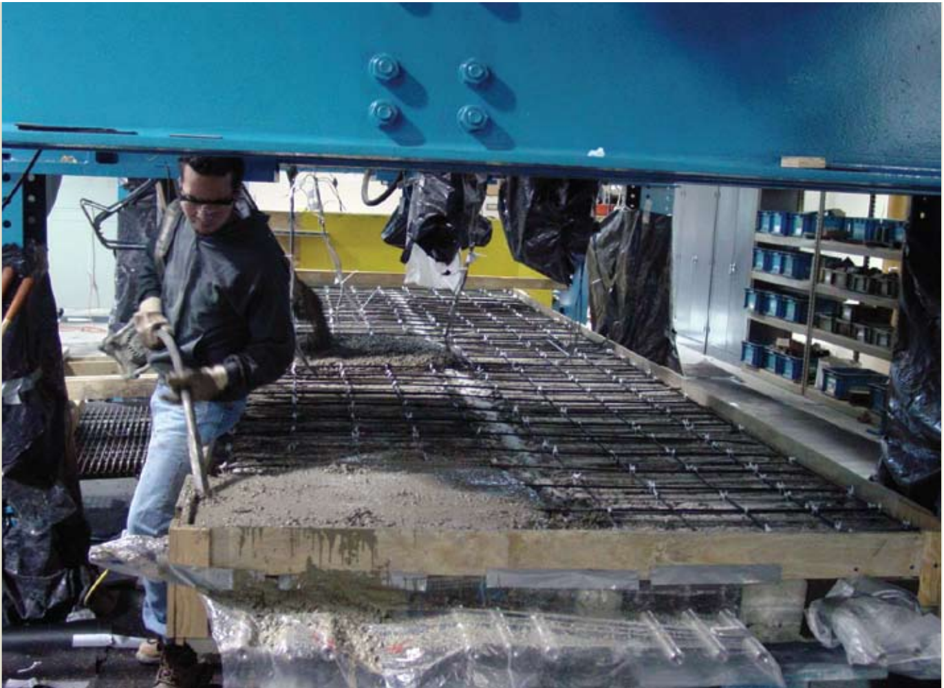
Figure 17. The concrete deck slab was placed over two adjacent box beams for one of the bridge models.
