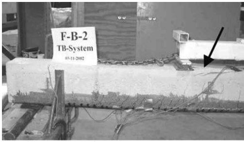
(a) Beam F-B-2 (concrete compression failure)
