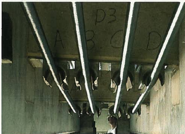
Fig. 6. Externally draped post-tensioning CFCC strands (looking from below DT beam).
