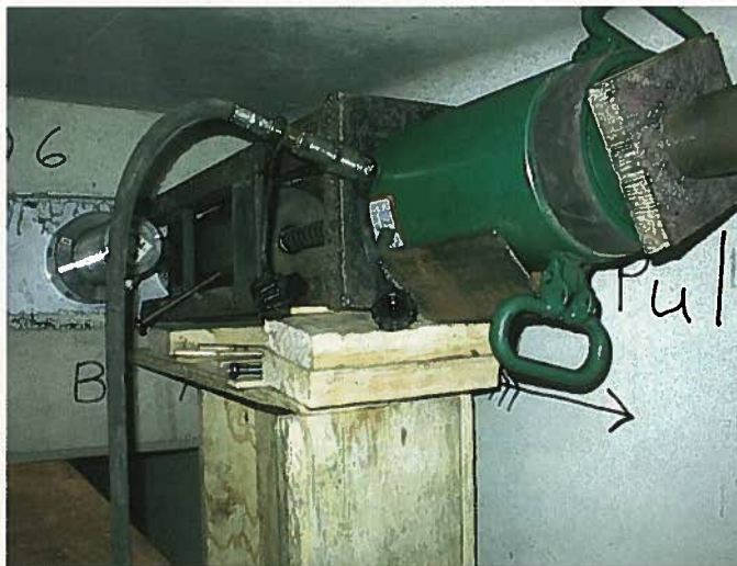
Fig. 8. Post-tensioning apparatus for a CFCC externally draped strand.
