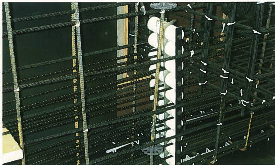
Fig. 3. Pretensioned CFRP Leadline™ tendons at roller hold-down location.
