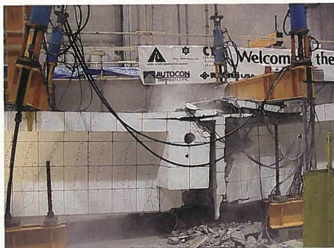
Fig. 16. Closeup of beam failure. External unbonded CFCC post-tensioning strands did not rupture.
