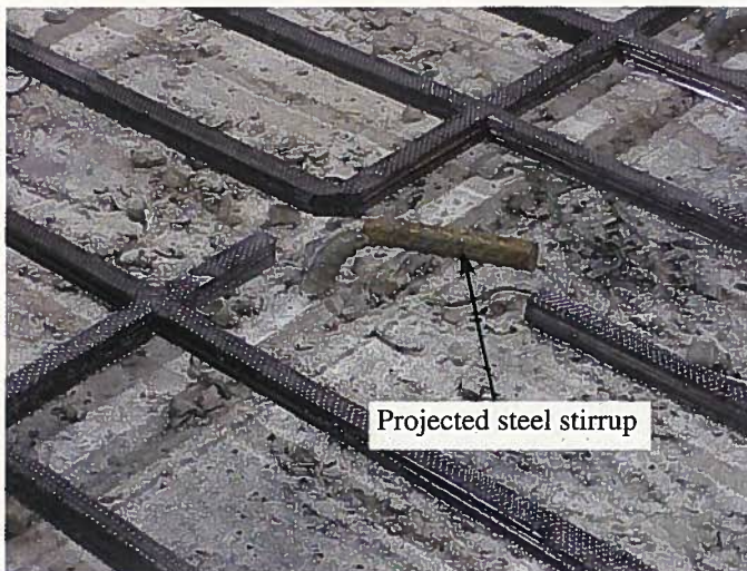
Fig. 9. NEFMAC reinforcing grid placed over the flange top.
