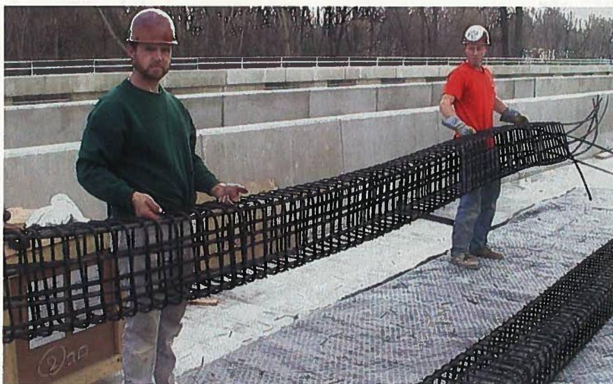
Fig. 18. CFCC reinforcement cage for top concrete barrier (under handrail).
