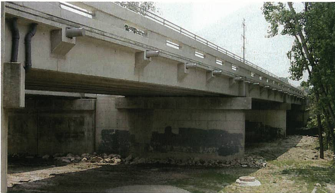
Fig. 13. Structure B completed and ready for traffic.
