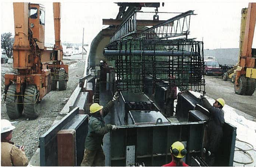
Fig. 6. Placement of non-prestressed CFRP reinforcement cage in single pan form.
