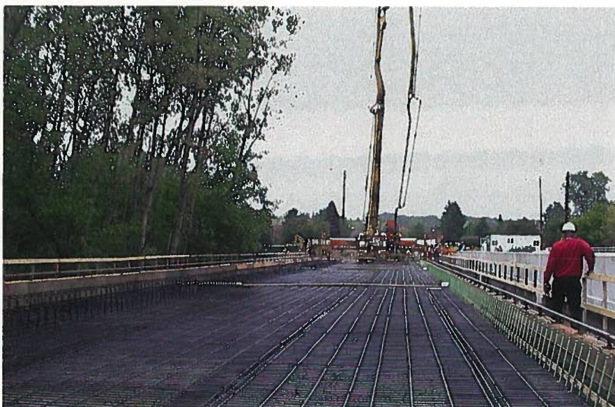
Fig. 17. NEFMAC grid placed over the flange of DT girders prior to placement of bridge deck slab.
