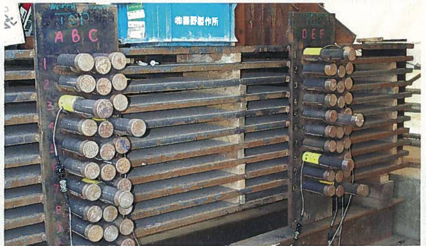
(b) Prestressing force measurements at dead end
