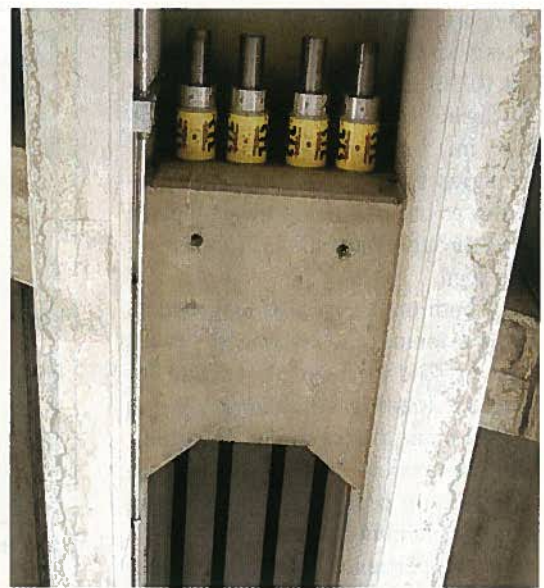
Fig. 10. Post-tensioning at the live end (left) and load cells installed at the dead end (right) for the longitudinal CFCC strands.
