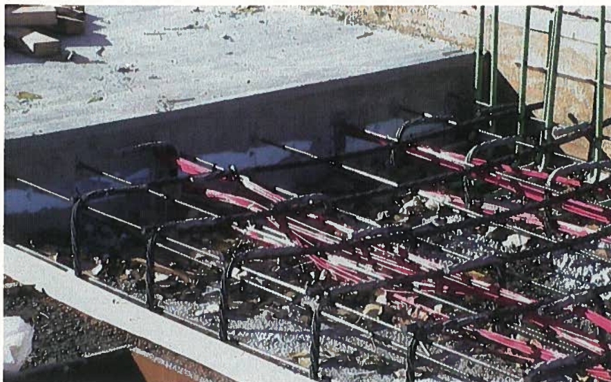
Fig. 20. CFRP Leadline and CFCC reinforcements for sidewalks.
