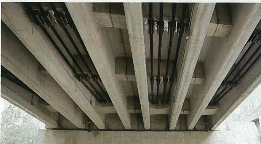
Fig. 12. Installed DT girders with external CFCC post-tensioning strands in place.
