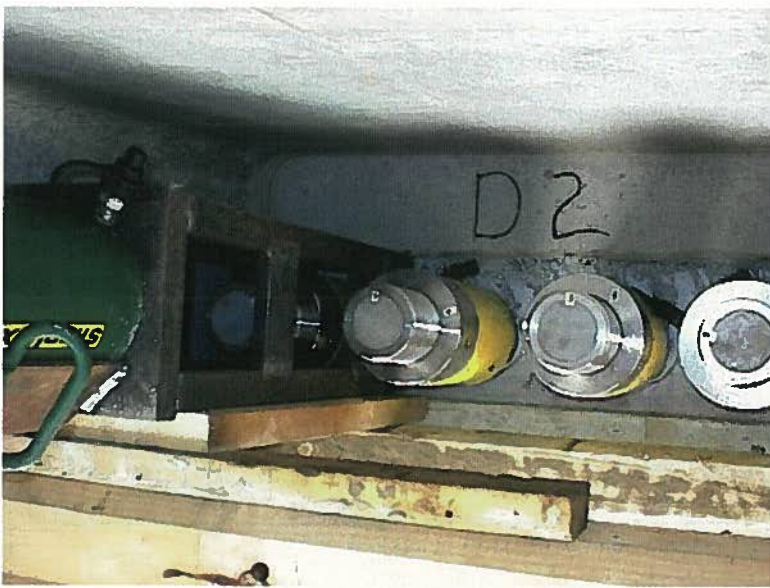
Fig. 10. Post-tensioning at the live end (left) and load cells installed at the dead end (right) for the longitudinal CFCC strands.
