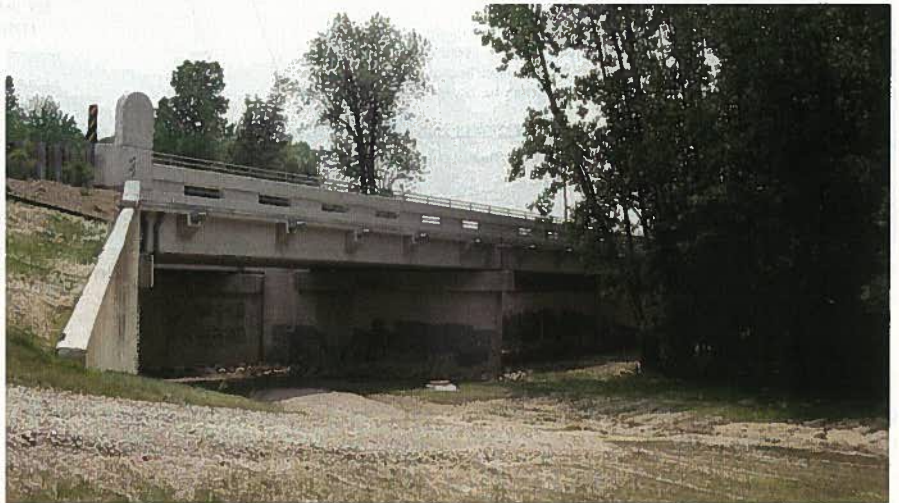
Fig. 1. (top photo) Bridge Street Bridge, Southfield, Michigan, looking south, with CFRP Structure B on the right. (bottom photo) Side view of Structure B.
