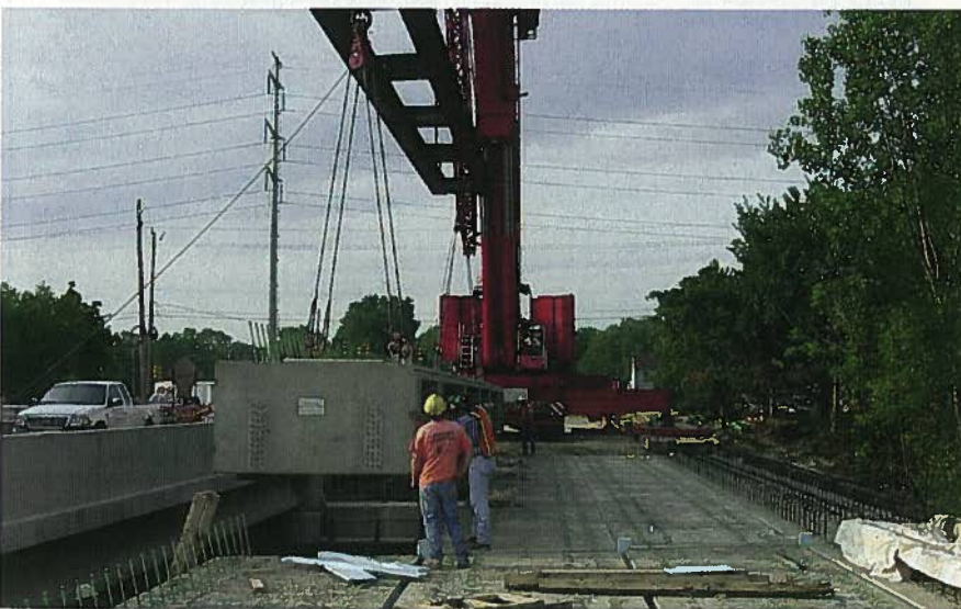
Fig. 11. Erection of DT girders at the bridge site.
