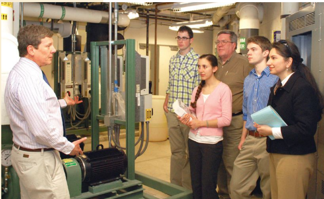
Associate Professor Robert Fletcher (left) and Architectural Engineering Director Filza Walters (right) discuss the geothermal system in the A. Alfred Taubman Student Services Center with architectural engineering students.
