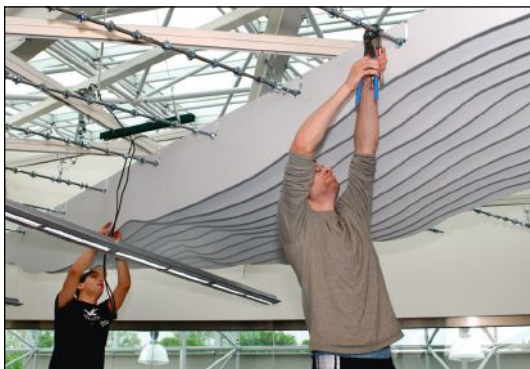
Pandush Gaqi (left) and Steve Kroodsma install baffles for the ceiling of the Welcome Center.
