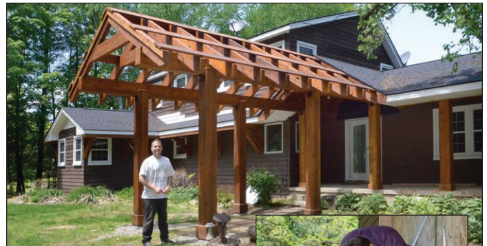
Jason Arnott designed this archway built with heavy timbers cut in the Northwest in the 1800s that were used as utility poles in Wisconsin.
