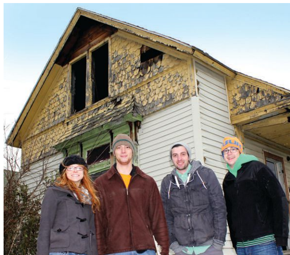
LTU students (L-R) Meaghan Markiewicz, Mike Paciero, Brandon Olsen, and James Sharp visit the house in Detroit that was later deconstructed to provide the lumber for a new structure.
